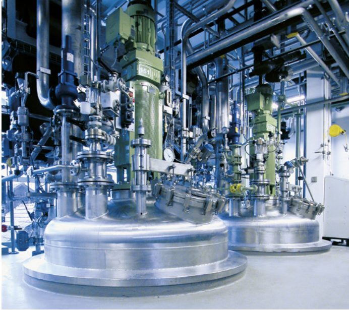
Chemical production facility at Siegfried in Zofingen
